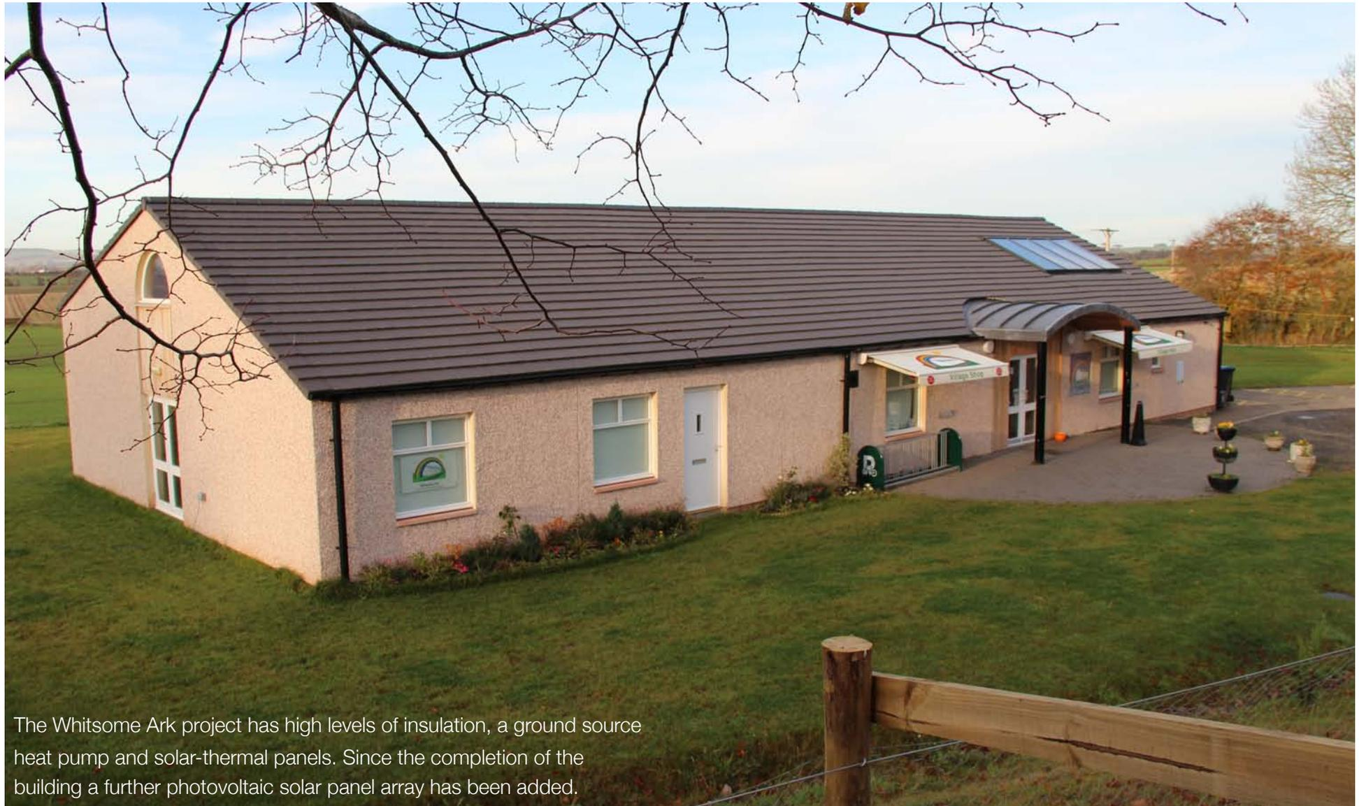
The Whitsome Ark project has high levels of insulation, a ground source heat pump and solar-thermal panels. Since the completion of the building a further photovoltaic solar panel array has been added.
